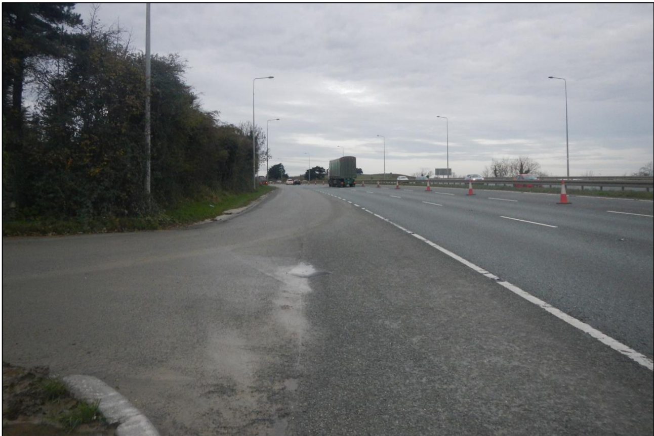
Figure 11.4: Looking West Along N7 from its junction with the Quarry Access.
